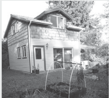
Second building, could be used for retail such as a garden center
